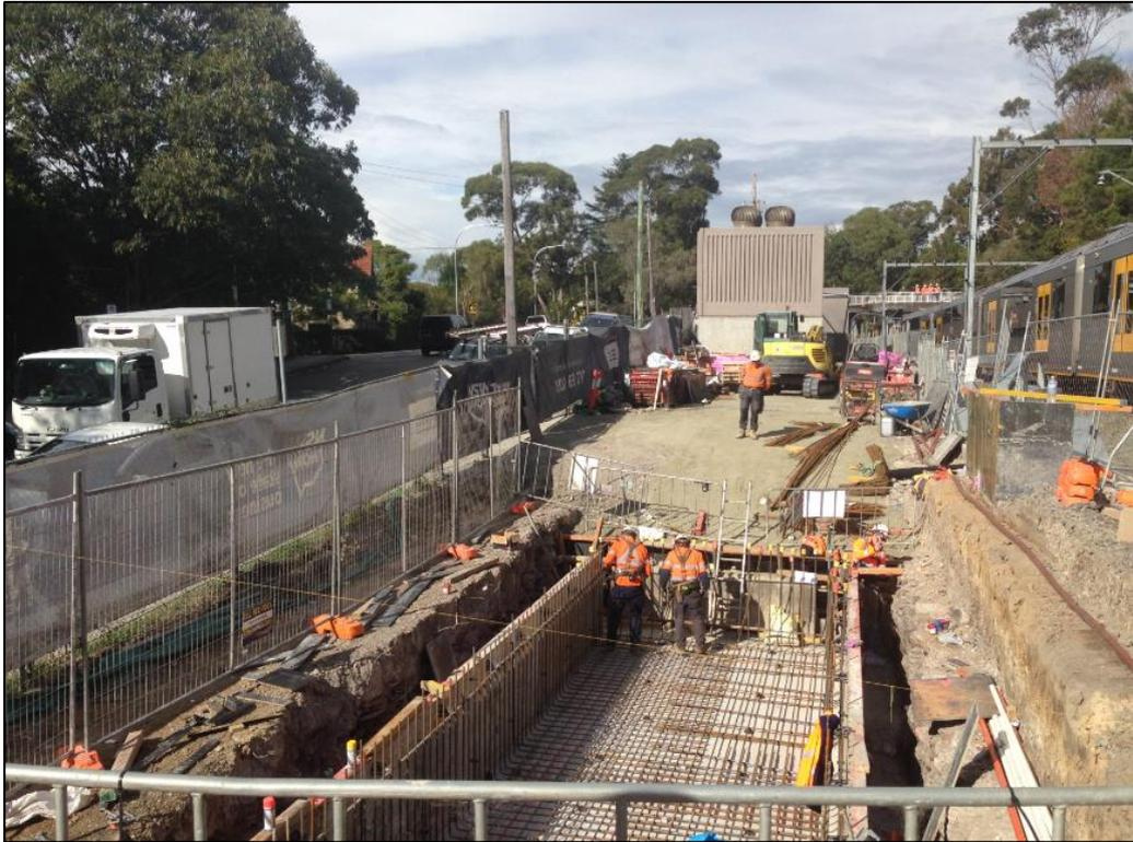
Figure 2 – Construction of the stormwater storage device and substation car park
