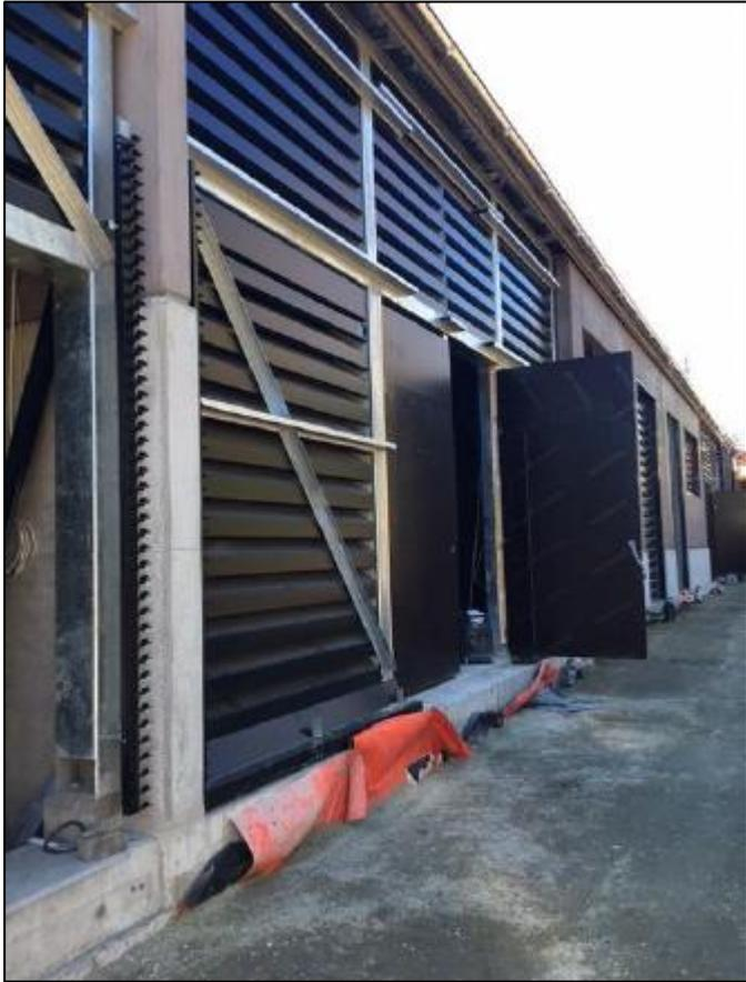
Figure 1 - Substation structure being erected and louvers installed
