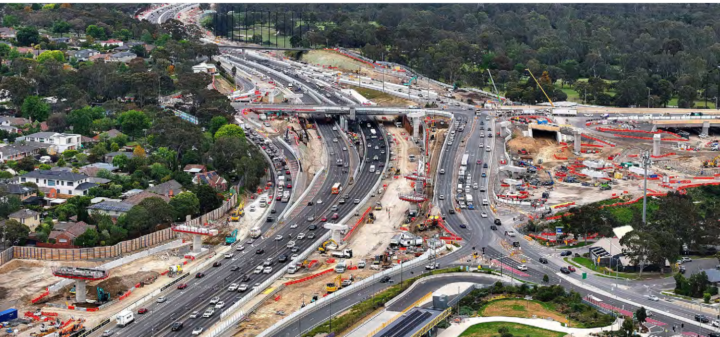
Eastern Freeway Upgrades – Burke Road to Tram Road project, Victoria, Australia
