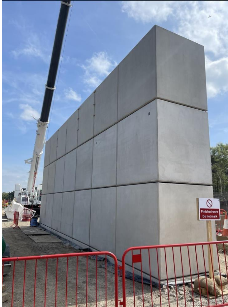
Finished Central Pier at Wisley Lane Overbridge
