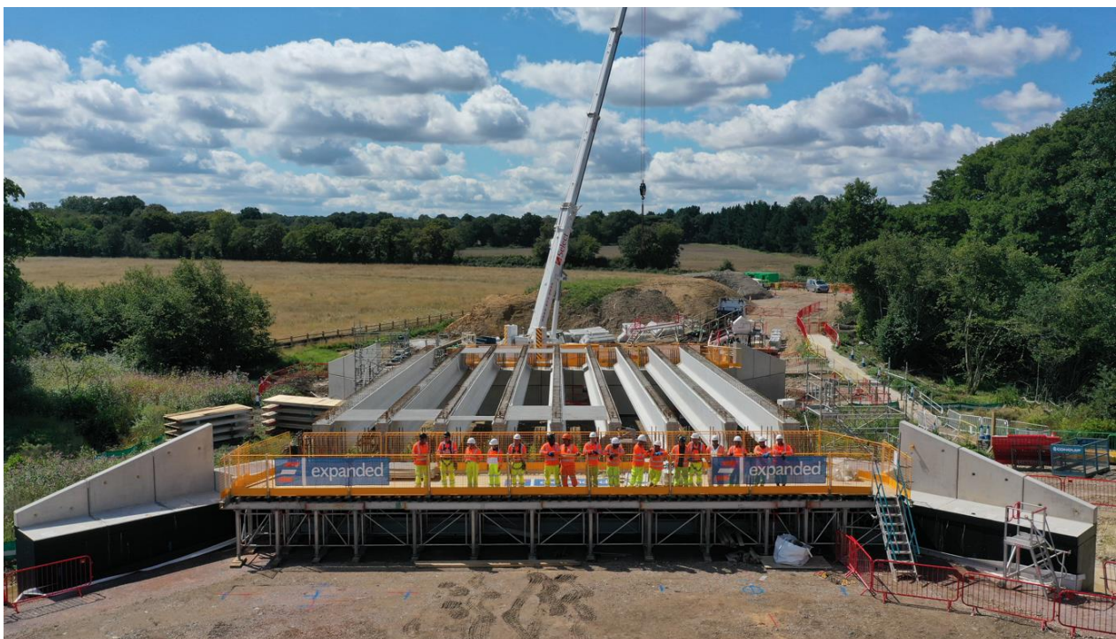
Beam installation over modular abutments at Stratford Brook Bridge
