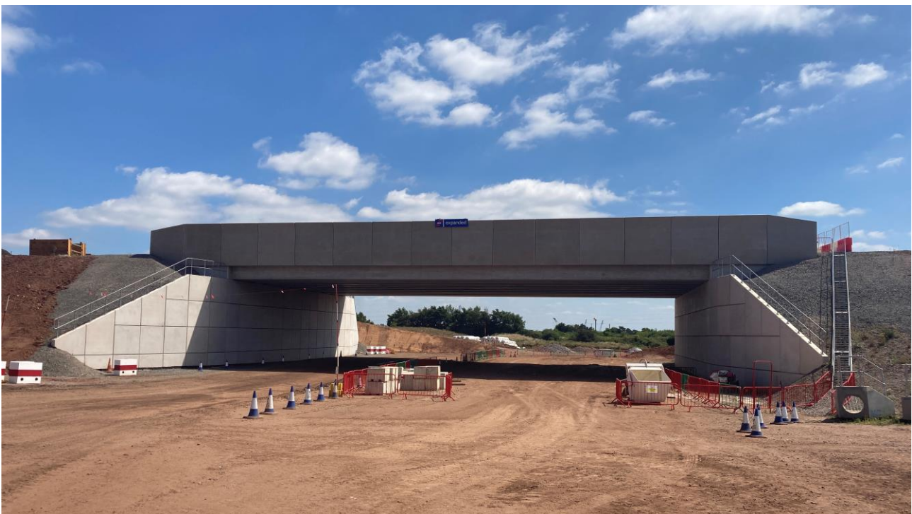
Completed HS2 Integral Bridge structure at Birmingham Interchange near Solihull
