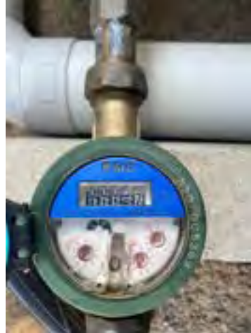
Image 2: Rainwater Harvesting Tank Meter
