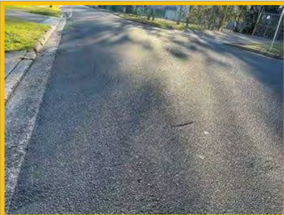
No. 038: 180m. gouge marks at layback to 12 Harris St extending to road centre
