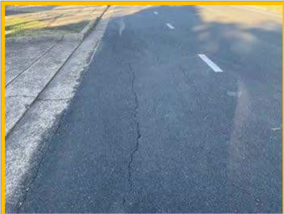
No. 057: longitudinal cracking and damage at entrance to 19 Harris Street (from 298m to 310m)
