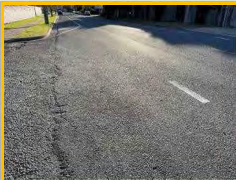
No. 093: 360m. Deterioration from the joint in materials leading to car park
