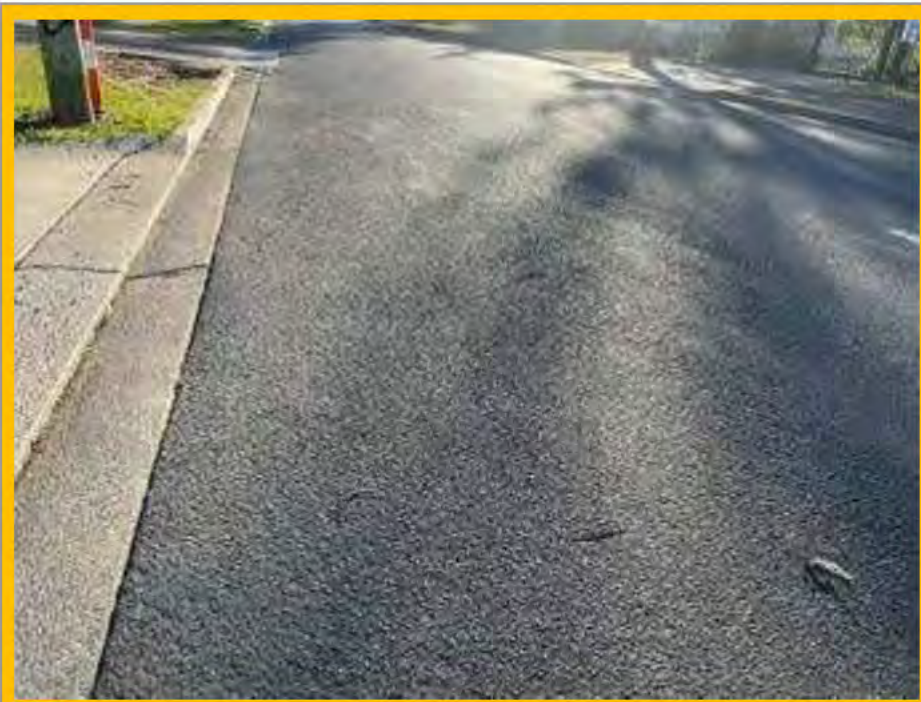
No. 017: varying gouge marks from 85-90m
