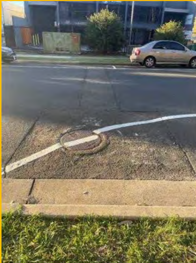
No. 115: depressions and cracking in road surface repairs extending across full width of road at 472m
