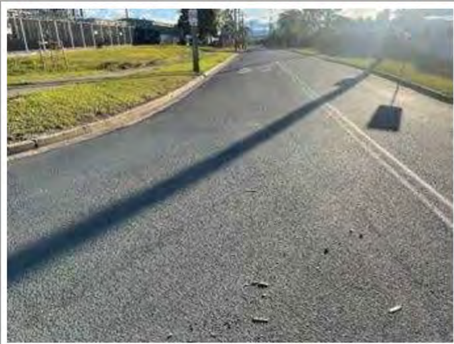
No. 001: Overview of Harris Street from the southeast corner at the intersection to Glossop Street. Survey began from this corner at 10m intervals which are marked for distance reference.
