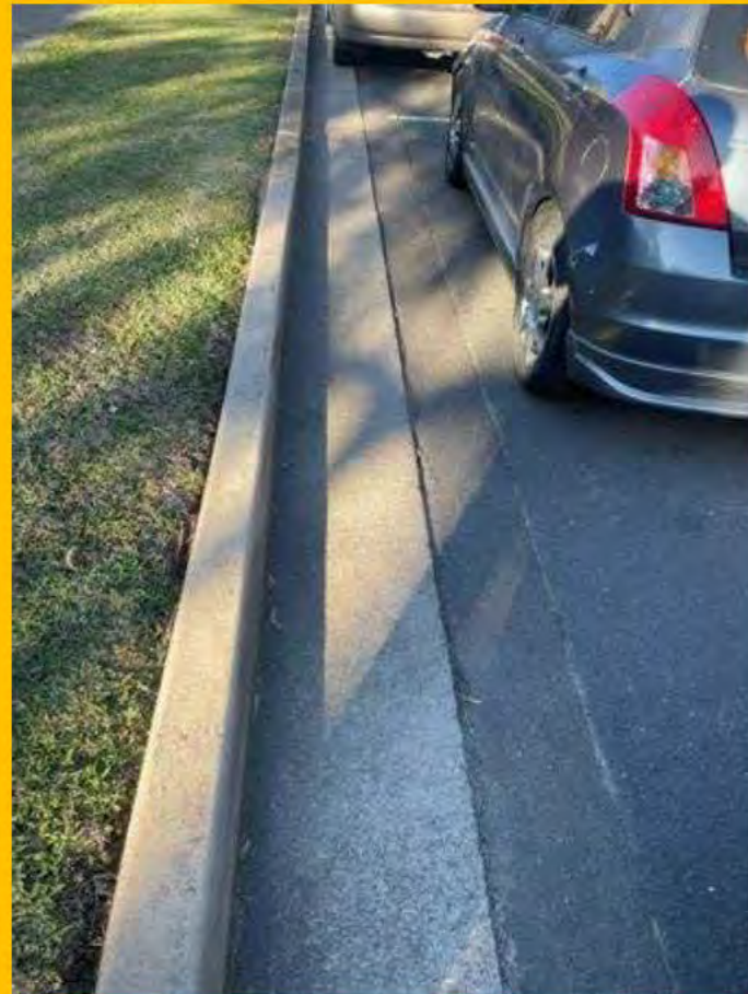
No. 016: 75m. Repairs to road surface at kerbline
