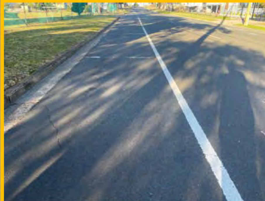
No. 048: cracking in surface at approx. 268m
