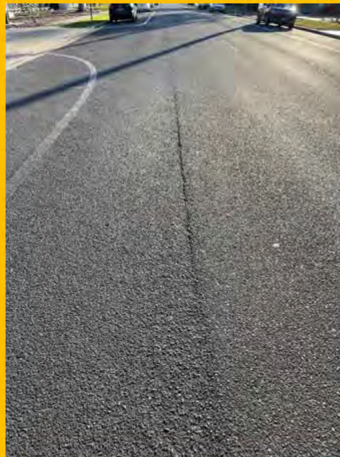
No. 104: crack commences at join in road materials at 415m
