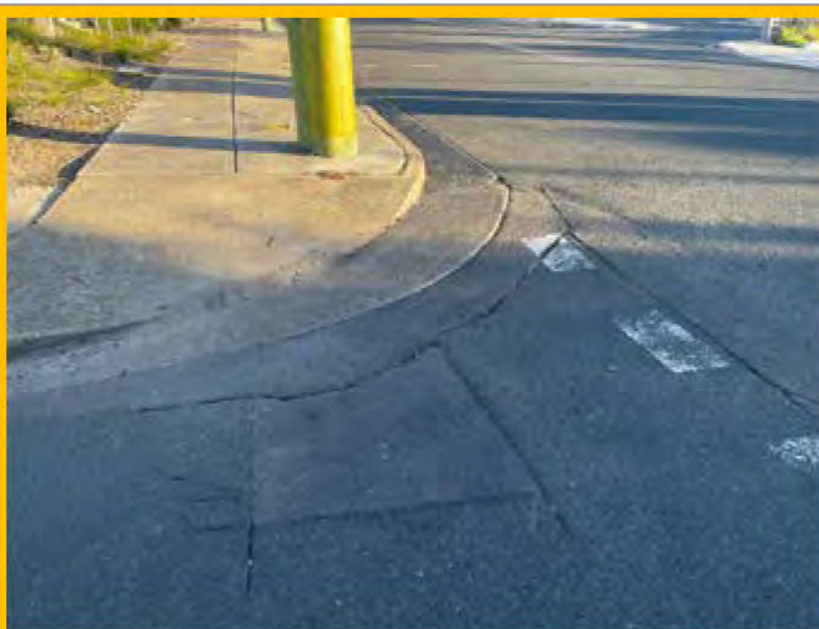
No. 129: depression and cracking to road surface at joins in road materials for previous repairs
