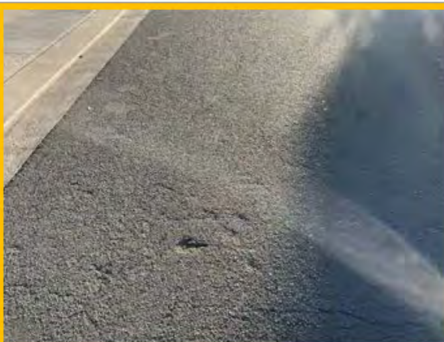
No. 117: gouging to road surface at 476m
