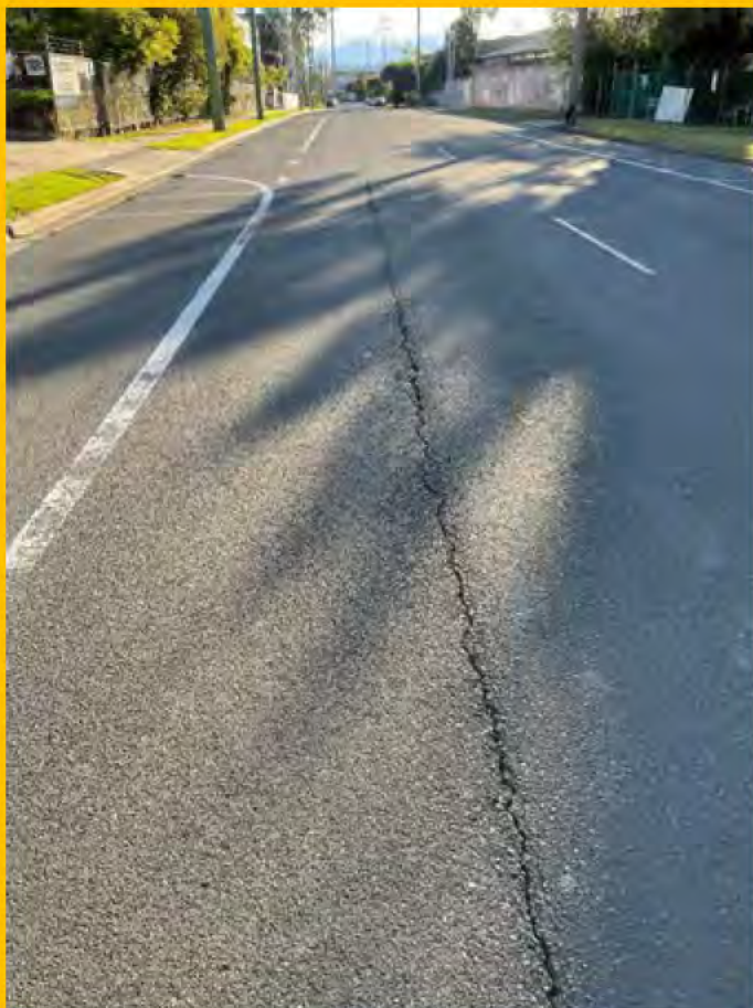
No. 055: continuation of crack in road centre
