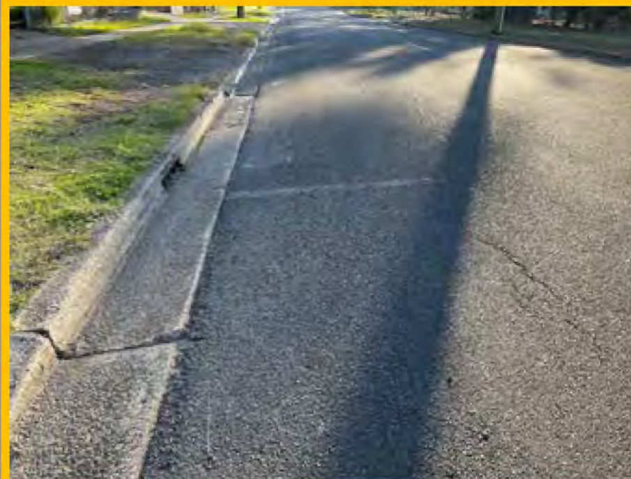
No. 034: 150m. cracking to road surface extends to approx. 151m
