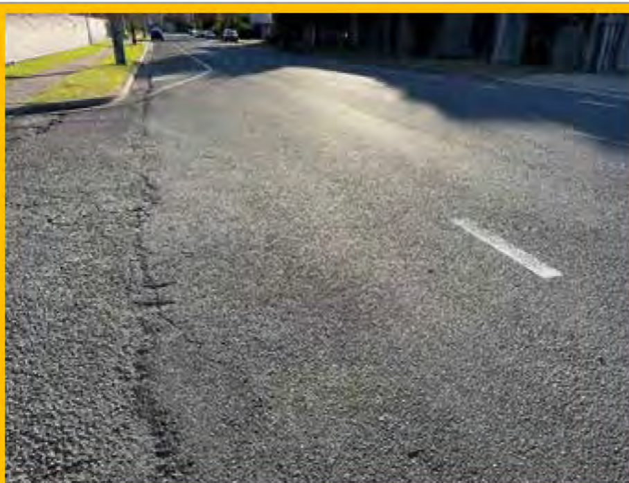
No. 093: 360m. Deterioration from the join in materials leading to car park
