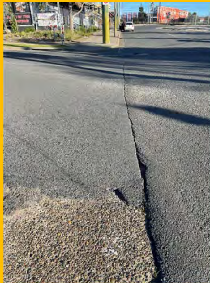
No. 002: Western end of Harris Street as it abuts Forrester Road. There is a crack at the join in road surfaces at this intersection and minor damage present.
