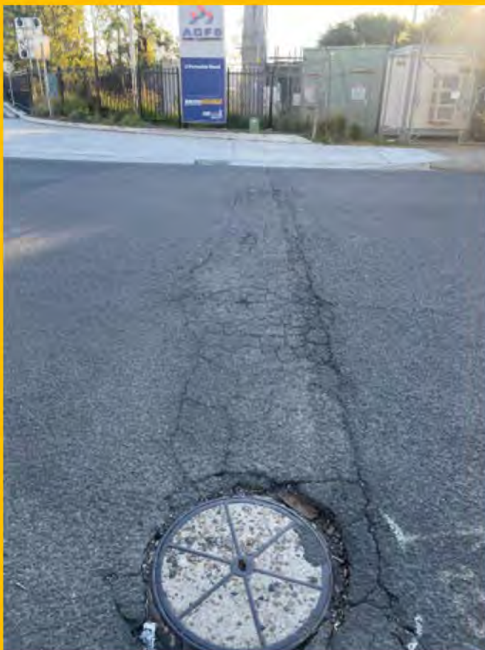
No. 001: Deterioration to road surface from intersection to Harris Street across full width of Forrester Road, viewed from Harris St.
