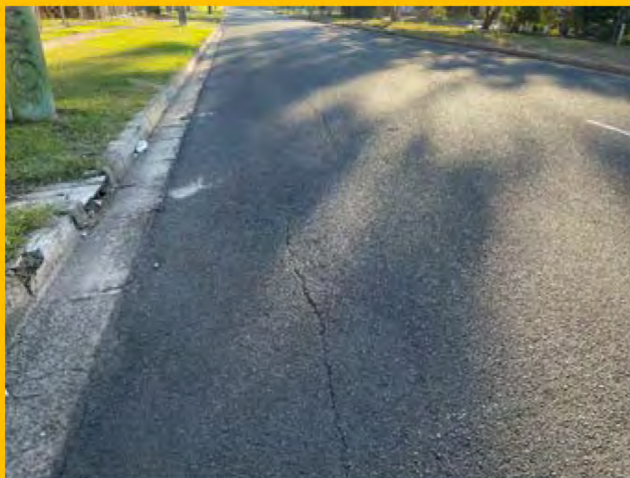
No. 025: continuation of cracking from 110-120m
