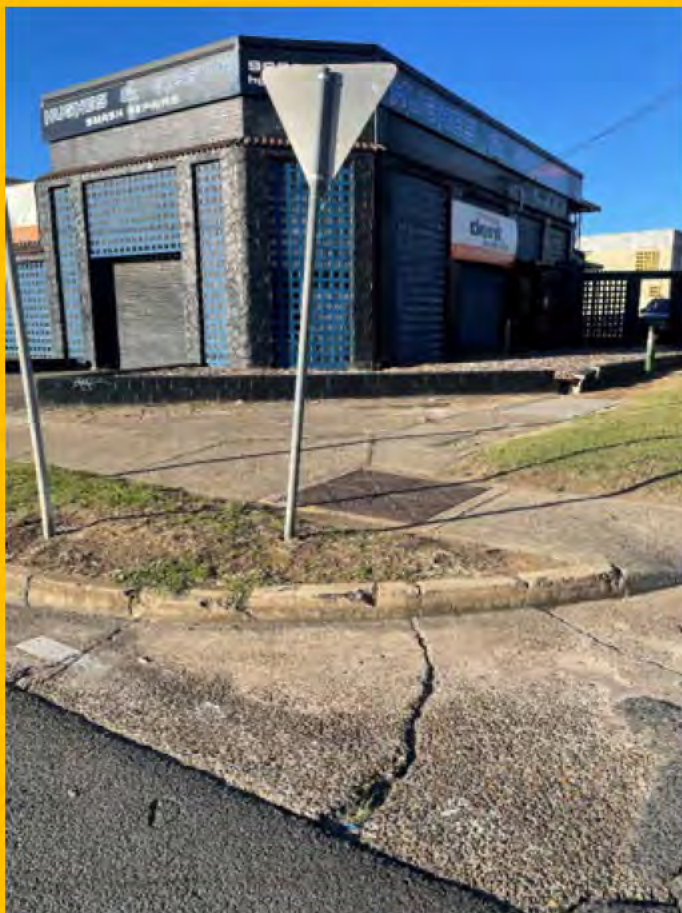
No. 003: View of building and footpath area on the northwest corner. The layback and kerbing are cracked and damaged
