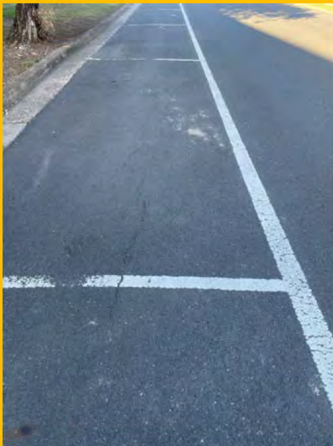
No. 025: Longitudinal cracking in road surface from approx. 135m to 140m
