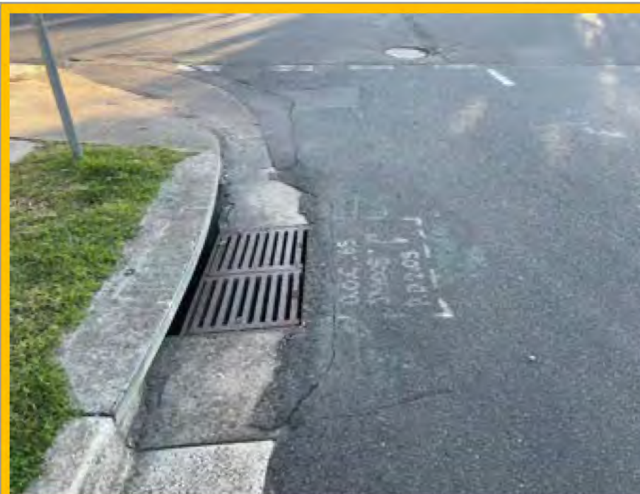
No. 128: cracking to road surface parallel to stormwater drain and at joins in road materials for previous repairs
