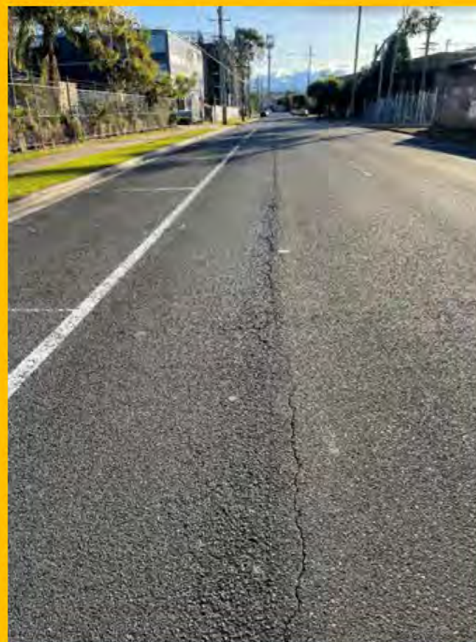
No. 074: cracking in road joint materials commences at approx. 297m
