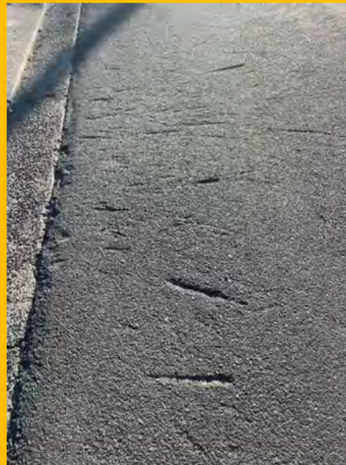
No. 030: gouge marks at 8 Harris St
