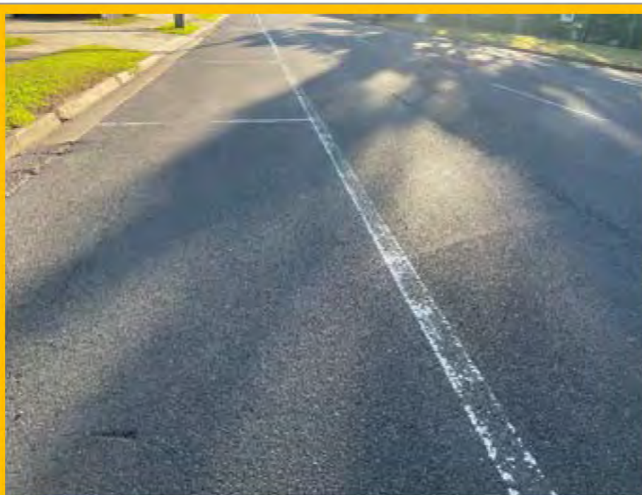
No. 053: continuation of crack in road centre. Minor gouging in parking bay at approx. 245m
