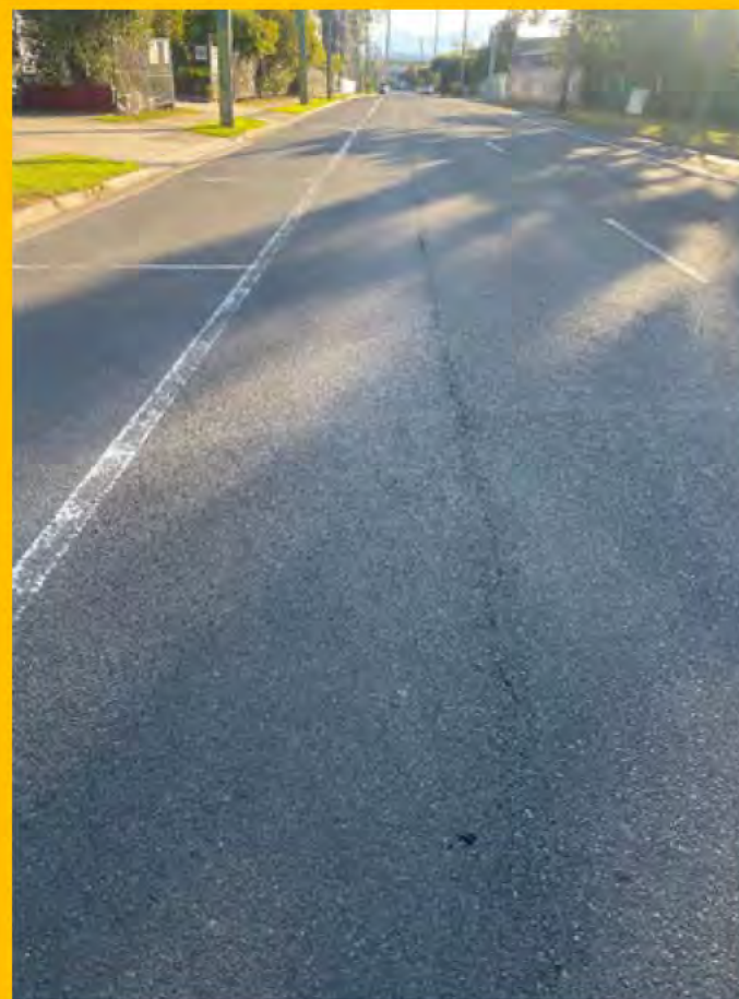
No. 052: longitudinal crack in road centre at join in materials commences from approx. 240m and continues through to approx. 290m
