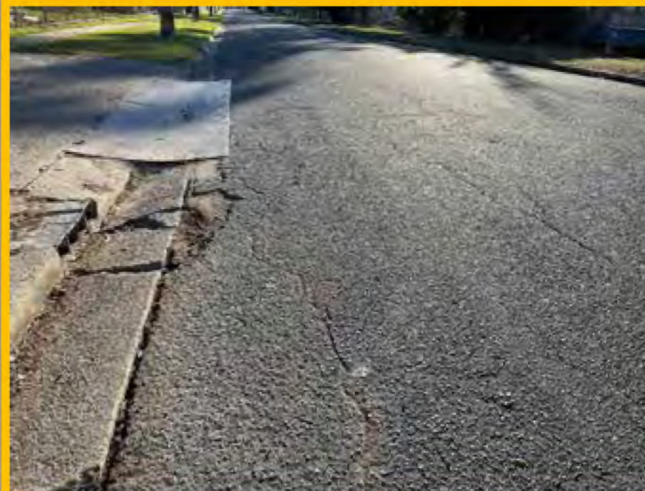
No. 020: 100m. continuation of cracking. Significant damage to road surface and layback at 6 Harris St
