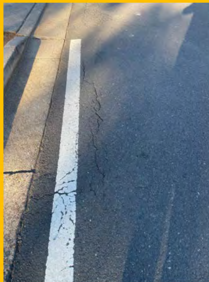
No. 066: continuation of cracking leading to driveway
