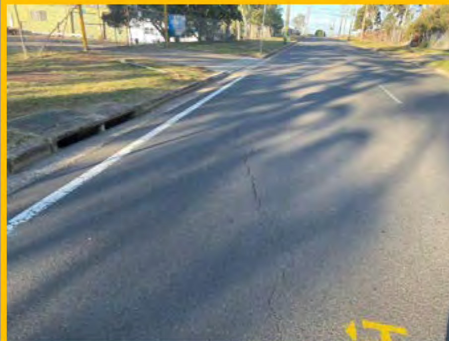
No. 064: cracking from centre of road leading toward kerblines at approx. 344m to 352m
