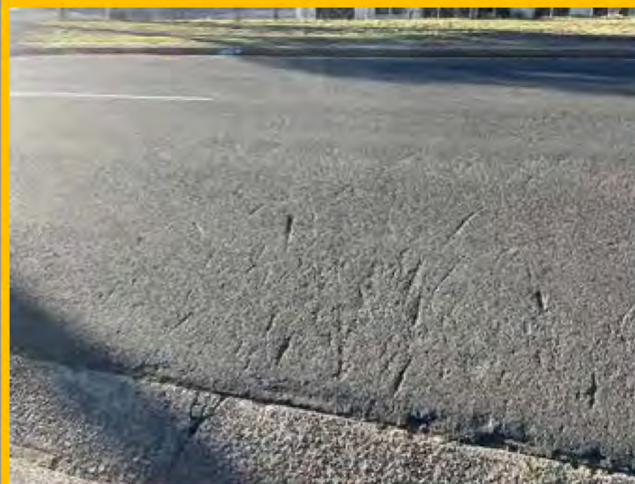
No. 032: gouge marks at 8 Harris St
