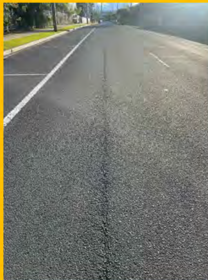
No. 068: continuation of crack in road centre
