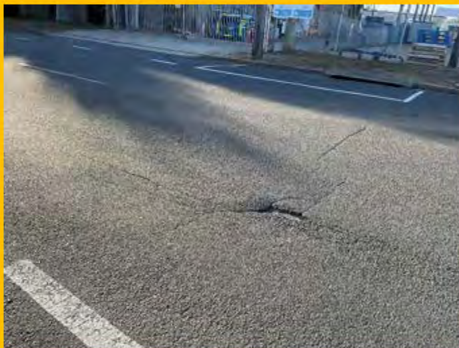
No. 091: damage and surface cracks at 355m
