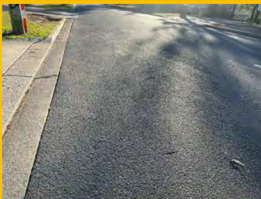
No. 017: varying gouge marks from 85-90m
