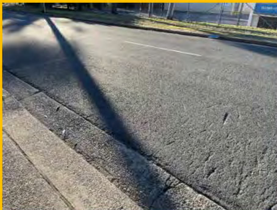
No. 033: gouge marks at 8 Harris St
