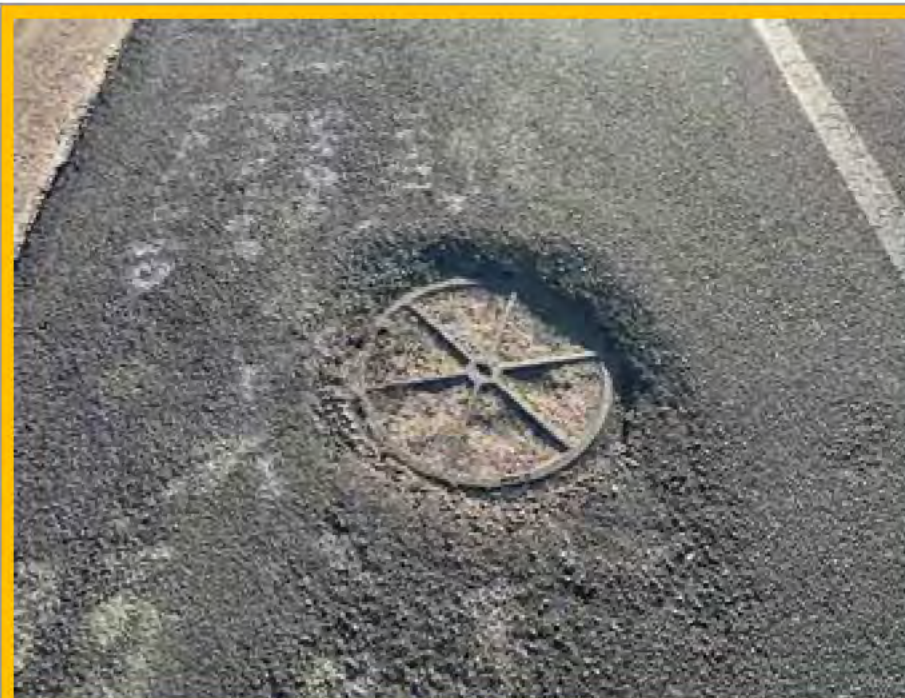
No. 100: depression at manhole cover at 395m
