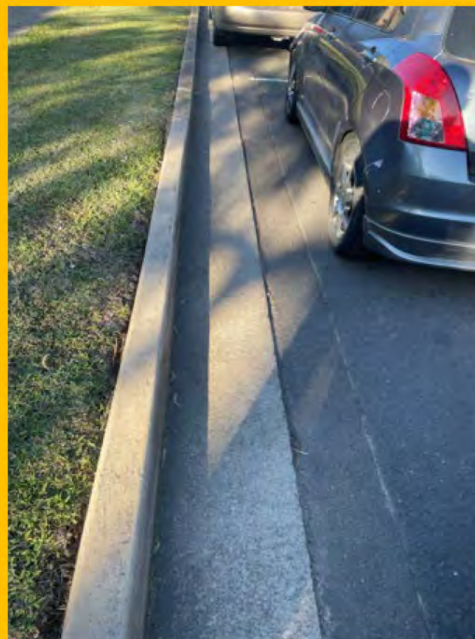
No. 016: 75m. Repairs to road surface at kerblin
