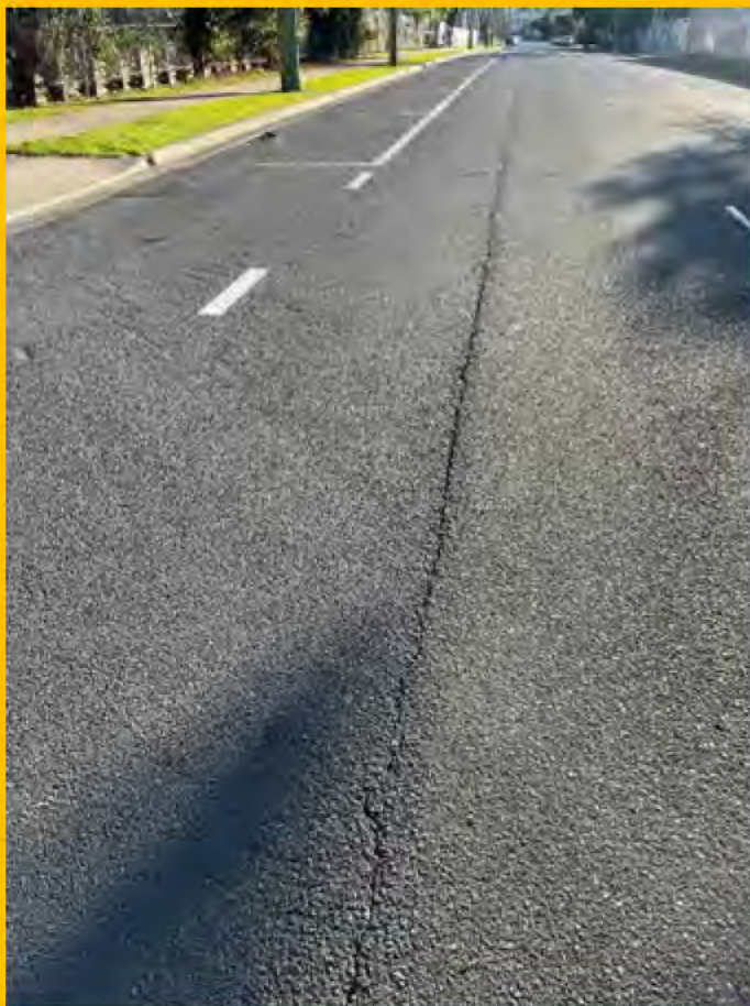
No. 063: continuation of crack in road centre
