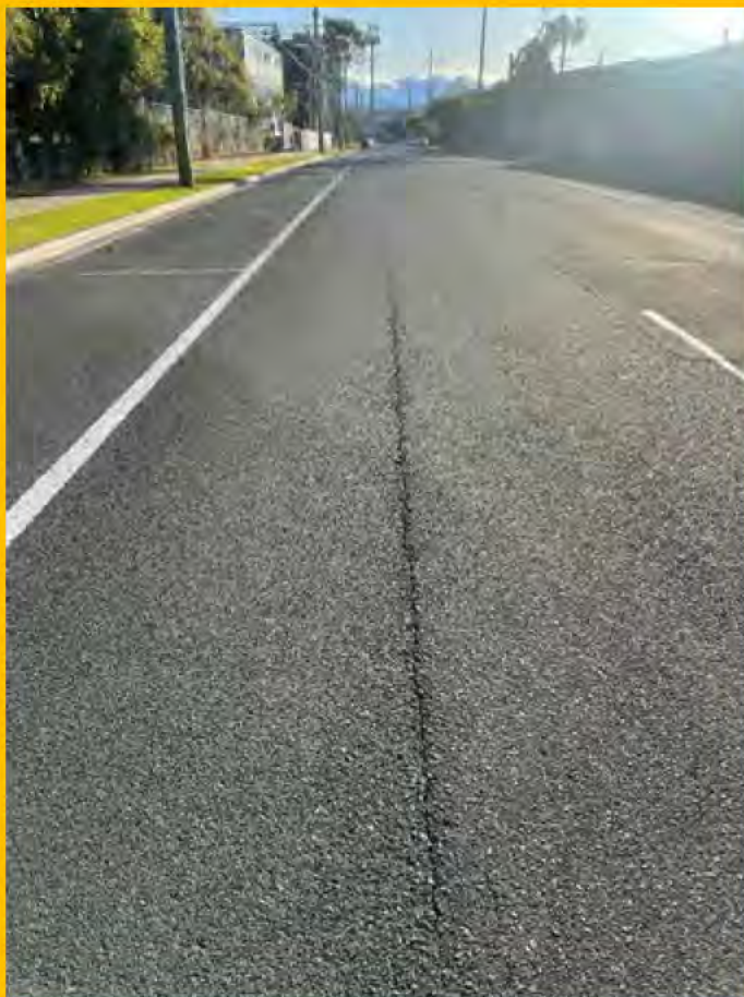
No. 069: continuation of crack in road centre
