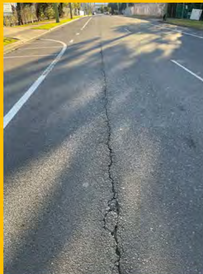
No. 058: continuation of crack in road centre
