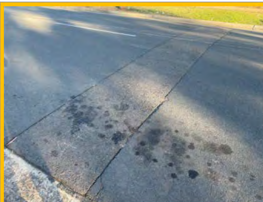
No. 082: Repairs to road surface across width of street at approx. 474m
