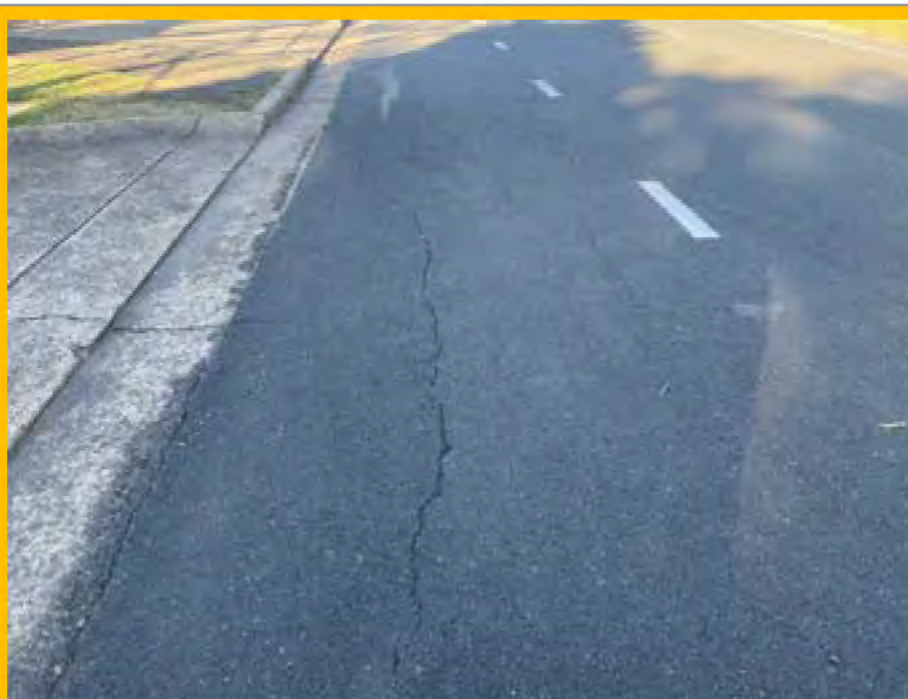
No. 057: longitudinal cracking and damage at entrance to 19 Harris Street (from 298m to 310m)
