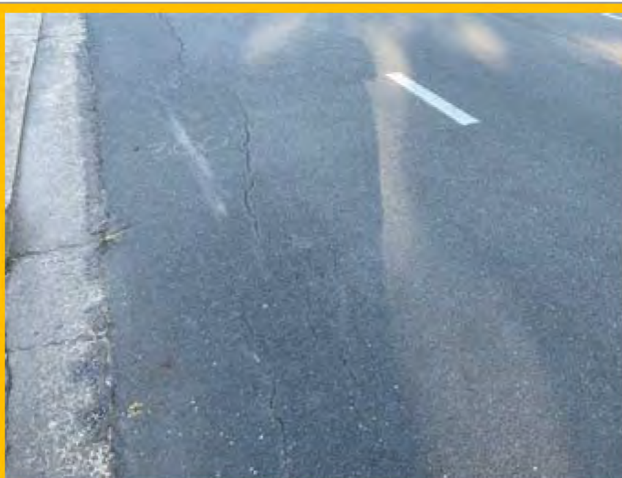
No. 055: longitudinal cracking from 298m to 310m
