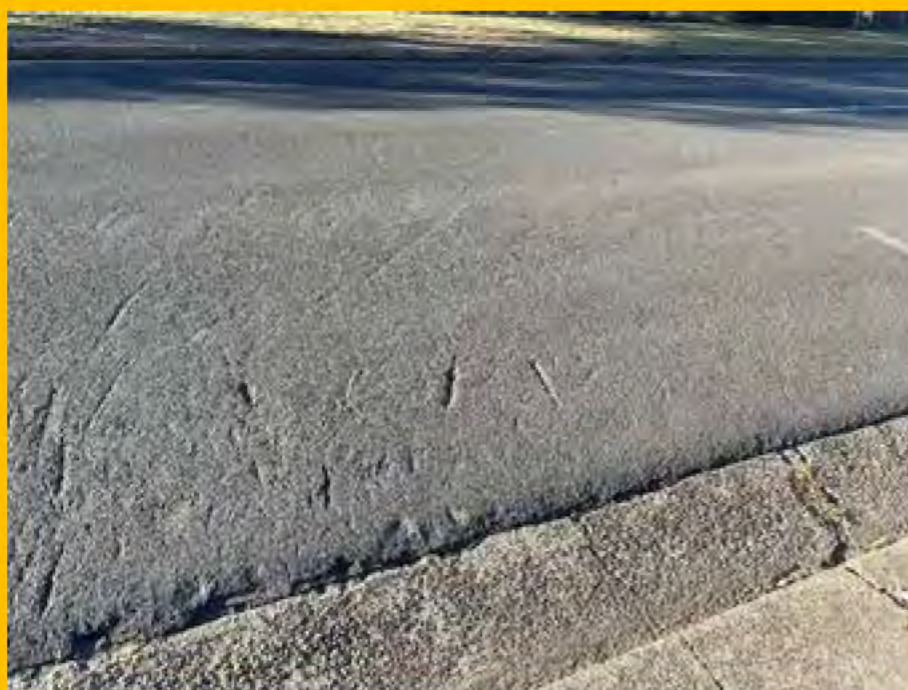
No. 031: gouge marks at 8 Harris St
