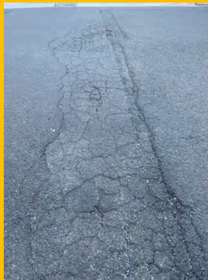
No. 004: deterioration and cracking of previous repairs to road surface
