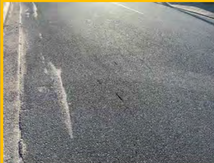
No. 006: general deterioration at 30m and beyond, and gouge marks at approx. 35m
