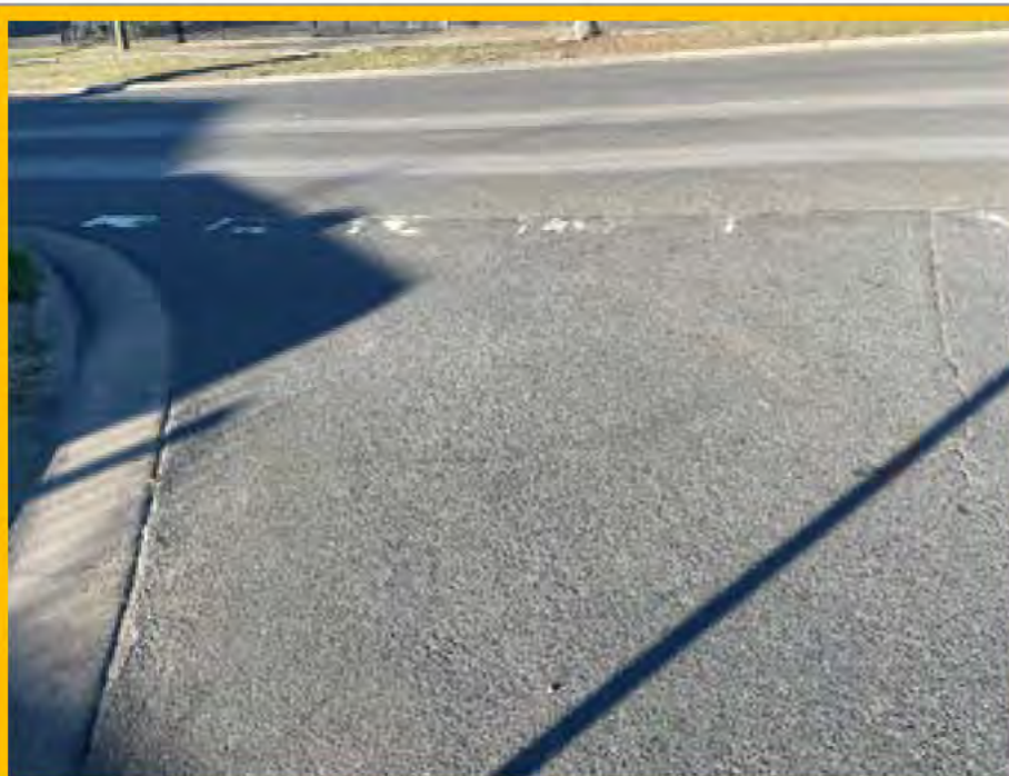
No. 091: longitudinal cracking commencing approx. 3m from intersection at Glossop St
