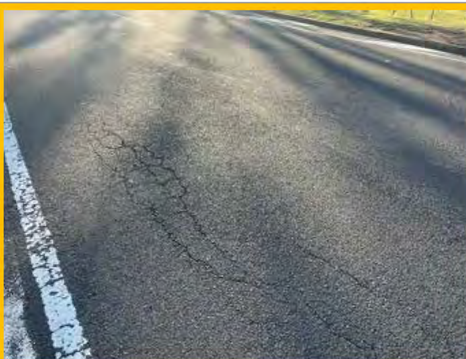
No. 045: cracking and deterioration of road surface from 210m to approx. 217m
