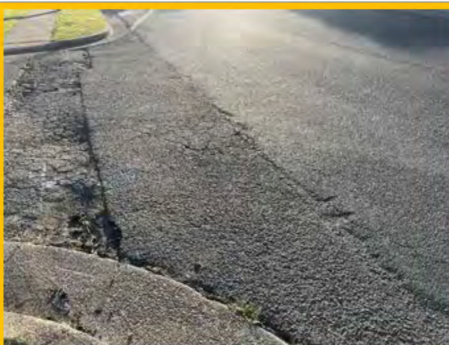
No. 095: deterioration of road surface repairs
