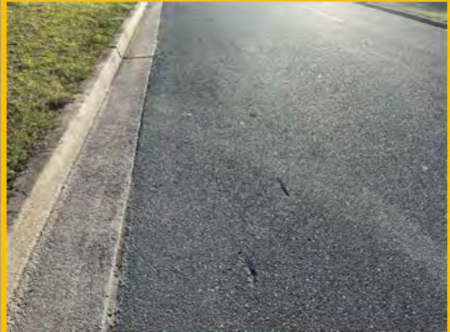
No. 008: gouge marks at 44m
